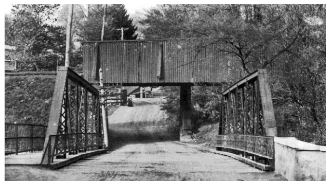
Two bridges of the past: the former 1898 Pratt Pony Truss bridge (rebuilt 2009) in the foreground crossing the White Clay Creek. In the background the bridge overpass on Landenberg road for both railroad companies, though primarily used by the Pomeroy Newark Railroad. (Courtesy NGTHC.)
