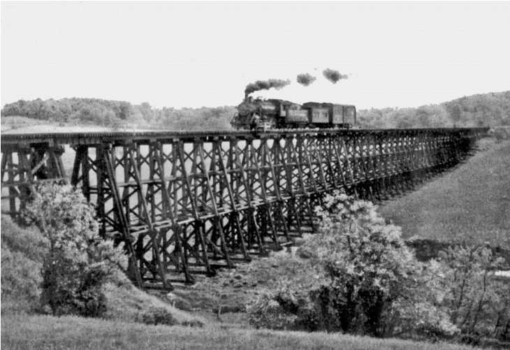
The Broad Run Trestle. Broad Run Trestle built for the Wilmington & Western Railroad. Erected 1873 and demolished during WW II. (Courtesy NGTHC.)
